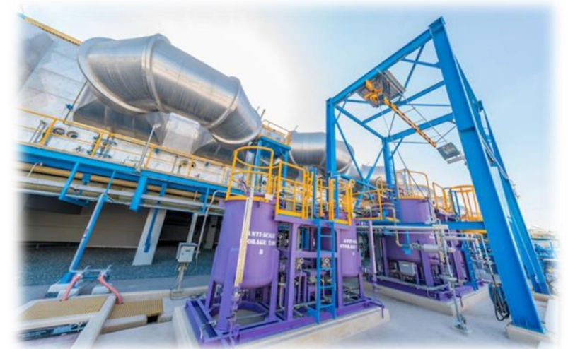
Facility E IWPP – Upcoming 2.4 GW / 110 MiGD project in Ras Abu Fontas.
